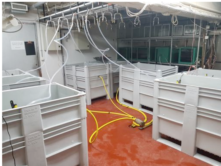
Figure 17: TZS Indoor mesocosm system
